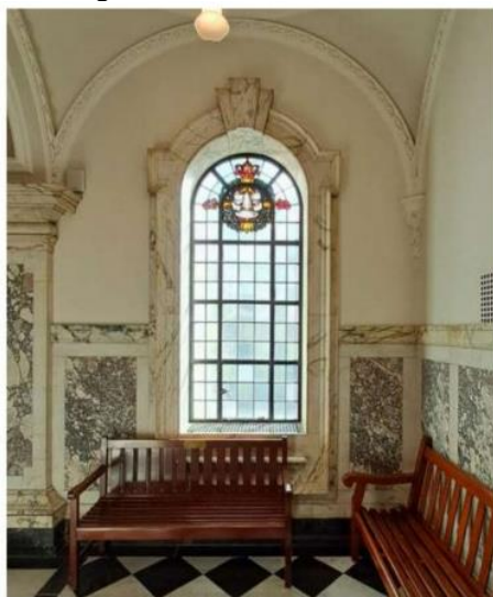
fig 1.1 & 1.2 - Internal views of existing stained glass windows to be removed, set into wooden crates and placed in storage
